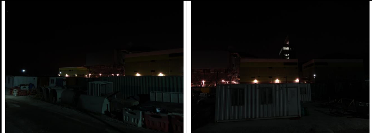
The lighting during night-time working is confined within the working area within the site boundary. Periphery area and the sensitive receivers are not affected by the lighting during night-time working.
