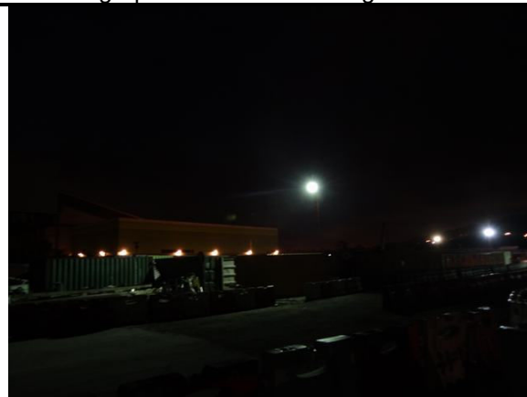
The lighting during night-time working is confined within the working area within the site boundary. Periphery area and the sensitive receivers are not affected by the lighting during night-time working.
