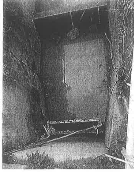
Photo 160714_003 (Main drainage channel) (Improved)
