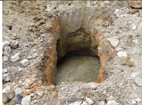
Photo 4: Groundwater was observed at the sampling pit
