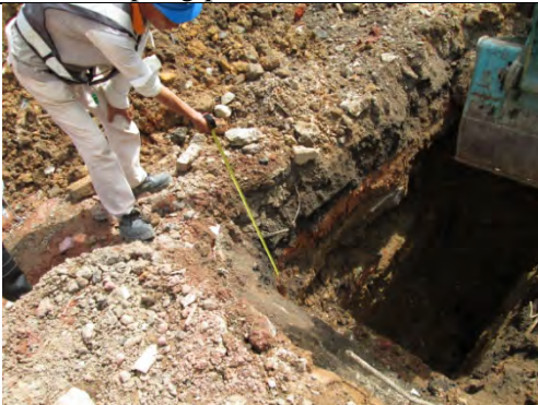
Photo 3: Sampling depth measurement
