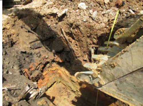
Photo 2: Sampling Pit excavation process
