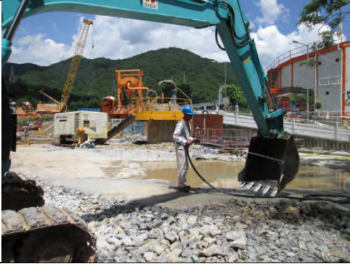
Photo 1: Perform an excavator decontamination
