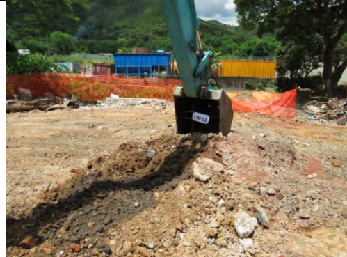
Photo 2: Sampling Pit excavation process
