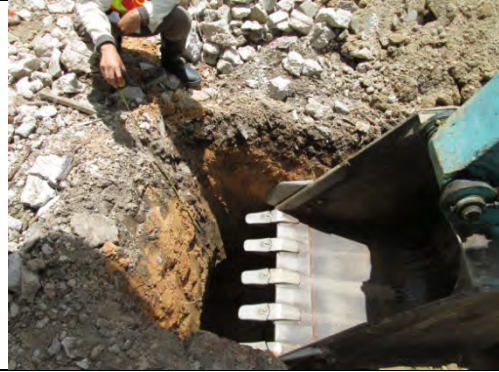
Photo 2: Sampling Pit excavation process
