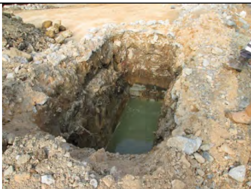
Photo 5: Groundwater was observed below existing ground level 2.4m bgl
