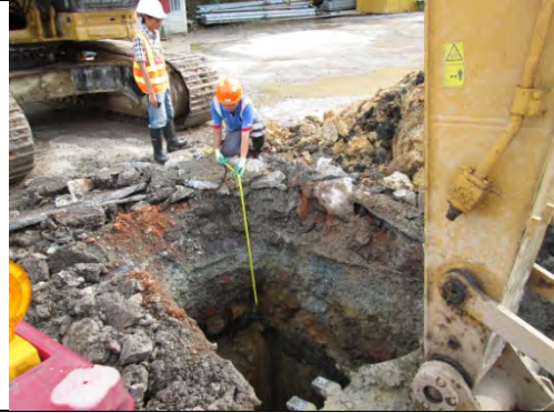
Photo 2: Soil Sampling Depth Measurement
