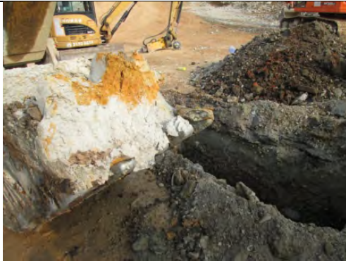
Photo 1: Sampling Pit excavated process
