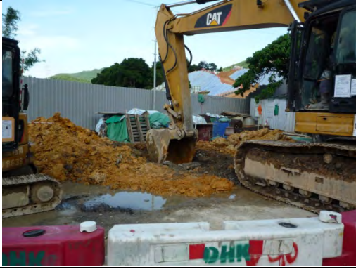
Photo 1: Sampling Pit excavated process
