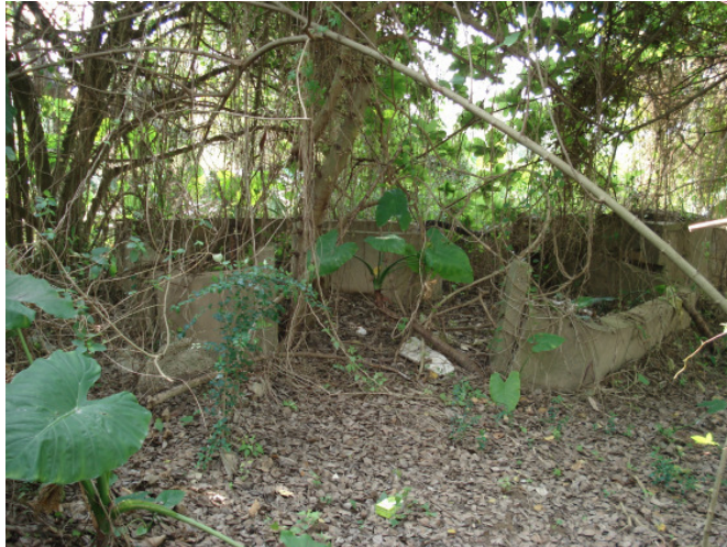
General view of the well
