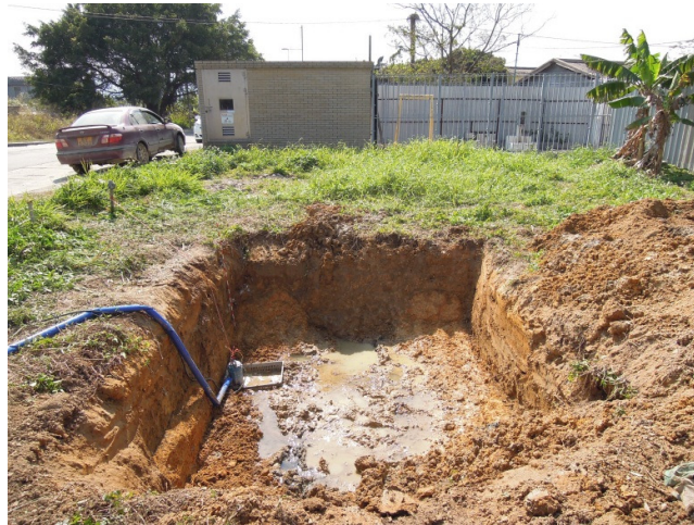
Overall view of M2 (view from north to south)
