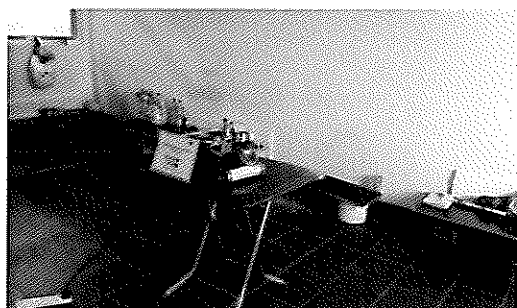
Store Keeper Office 2
