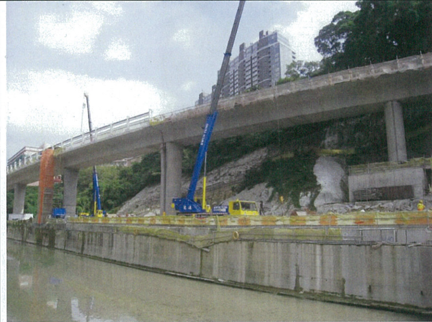
Plate 1. Existing rock slope near Viaduct Pier 12 and 13.
