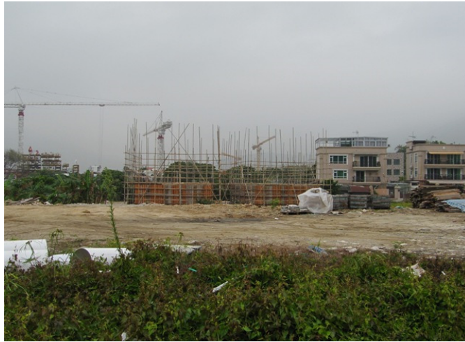
Plate 4 Non Project-related construction works at Point Count Location SSS-3/P6
