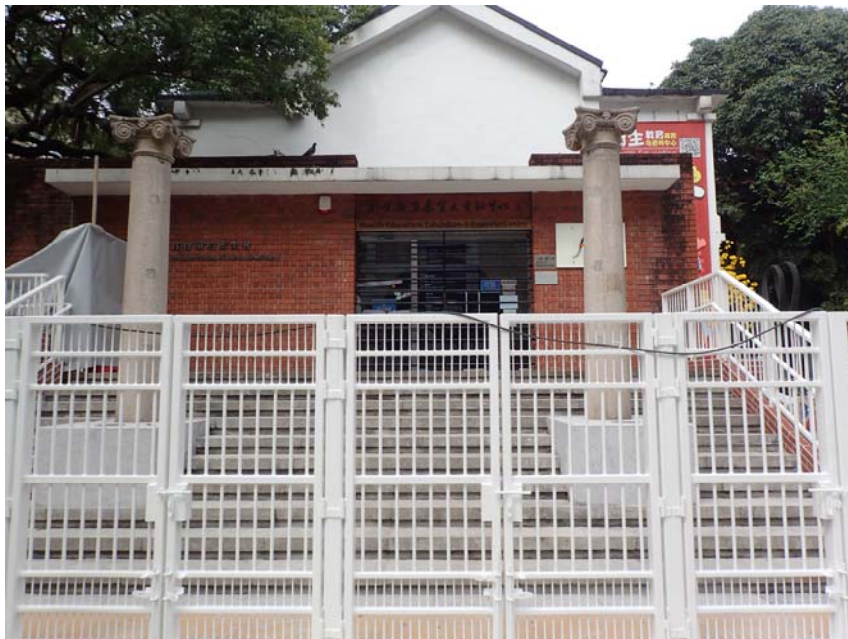
Photo record of the granite columns reinstated at Kowloon Park entrance
