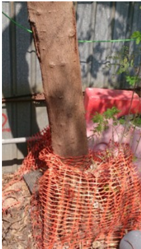
Photo 1a Construction materials were placed next to a tree which is located next to a red container
