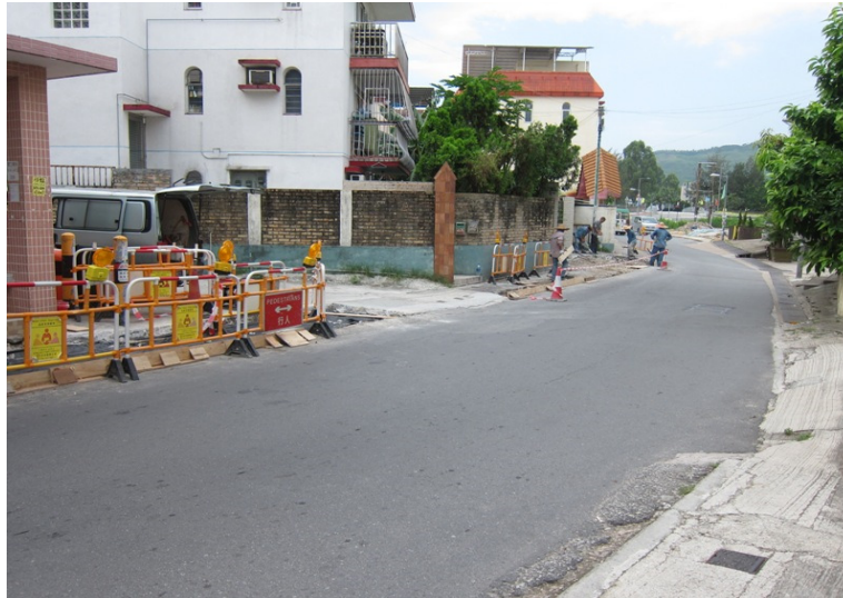
Plate 4 Non-project related Excavation Works near Point Count Location TPP-3/P1
