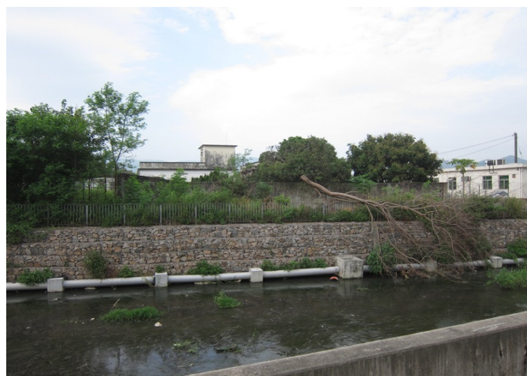
Plate 3 Felled tree along channel at Point Count Location TPP-1/P3
