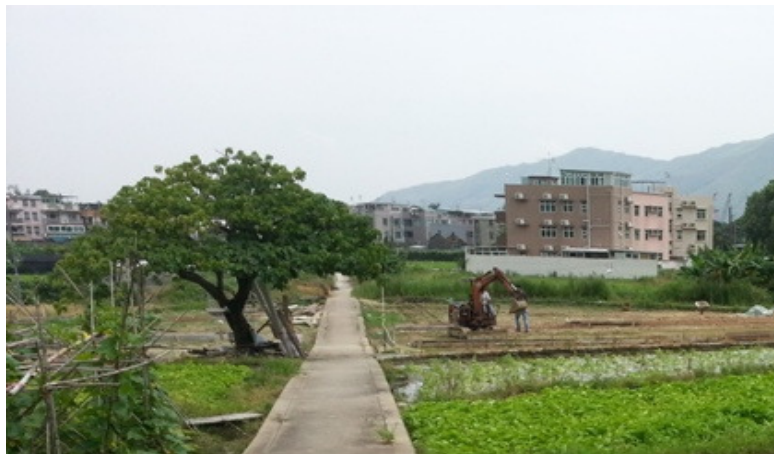
Plate 5 Non Project-related construction works at TUW-1/P4
