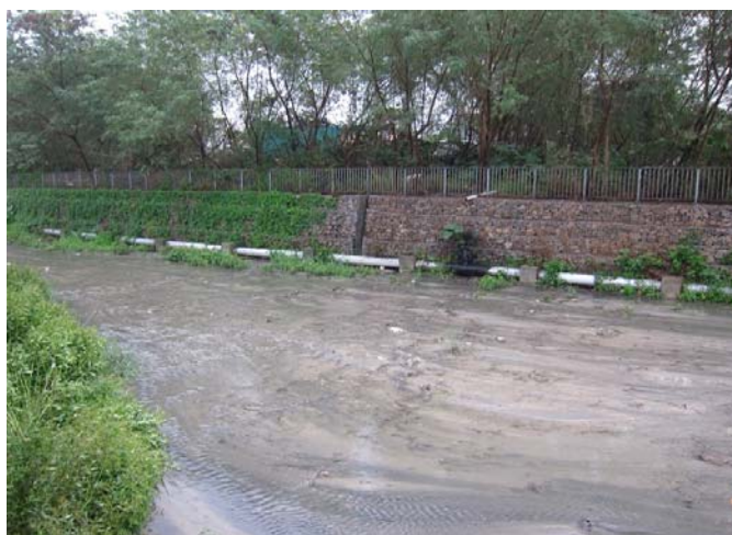
Plate 4 Vegetation removal on the gabion bank of KT5 at TPP-1/P3
