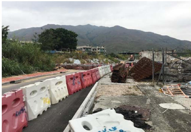
Plate 5 Hoardings and stockpiling materials along Point Count Locations TPP-1/P4
