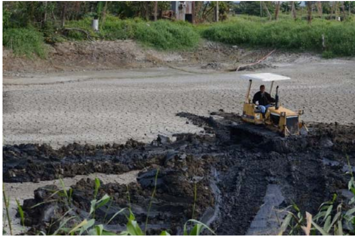
Plate 4 Pond was observed to be drained and site levelling works was being conducted at Point Count Location MPV-1/P3 (non-project related)
