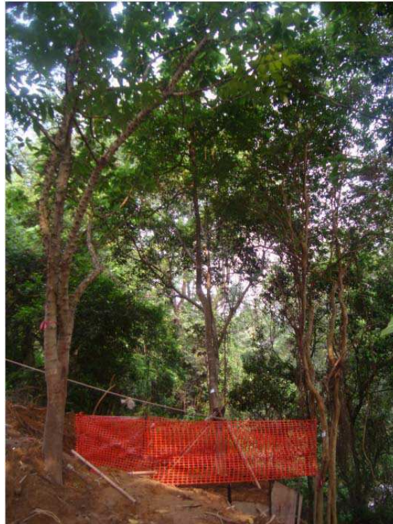
Photo 1 - Illustrative photo of 1.5m protective fencing
