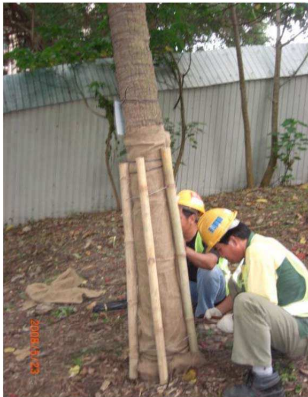
Photo 2 - Illustrative Photo of 1.5m high Tree Armoring Protection Method
