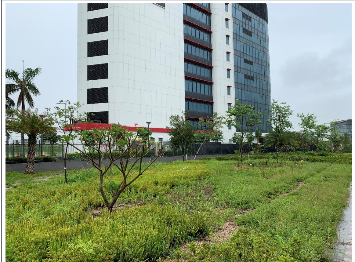
Photo 12: LCSD Area – Zone E
