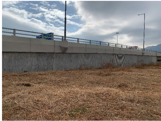
Photo F4 - The weeds were removed and maintenance is in progress.
