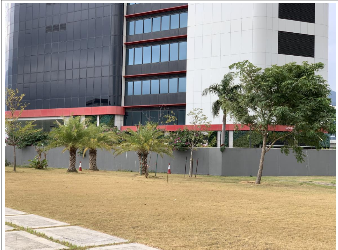
Photo 10: LCSD Area – Zone E
