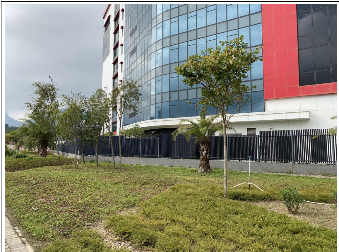
Photo 11: LCSD Area – Zone E
