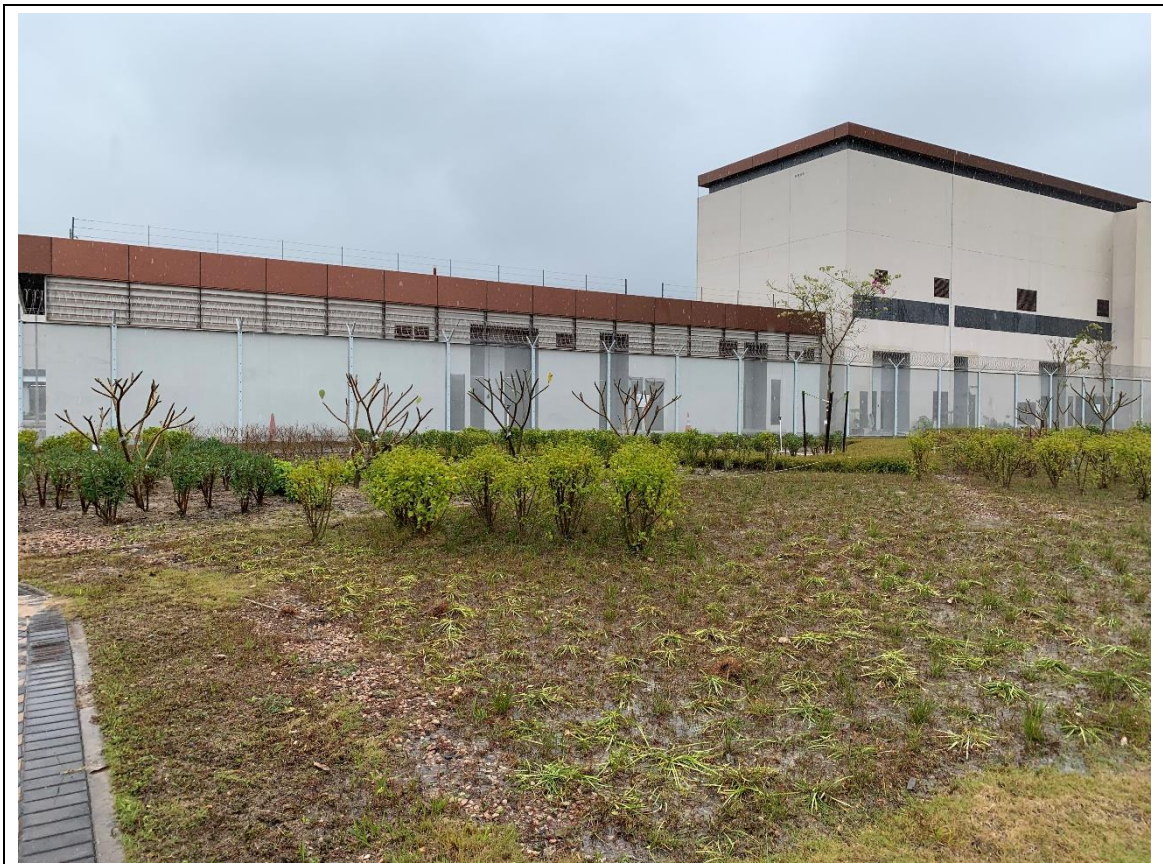
Photo 41: LCSD Area - Zone E
