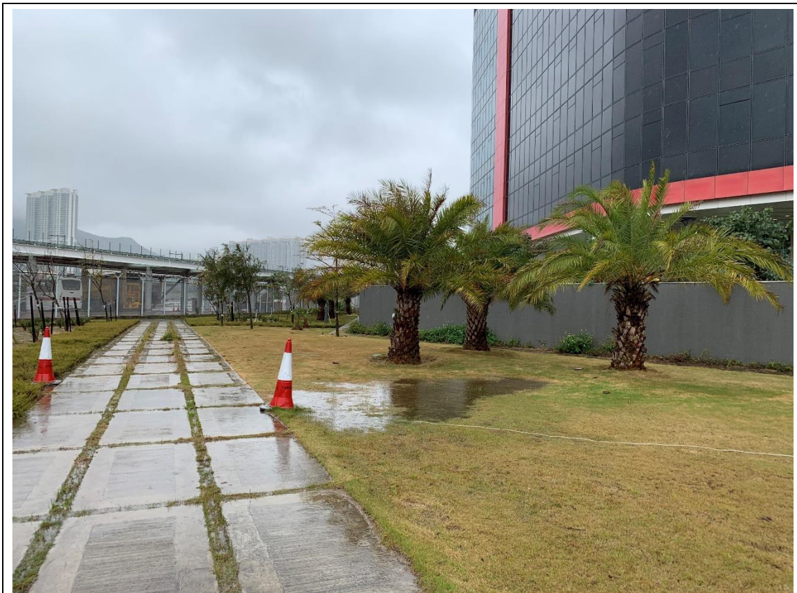
Photo 47: LCSD Area - Zone E
