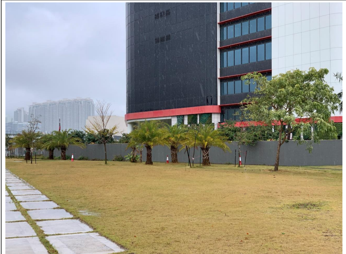
Photo 44: LCSD Area - Zone E
