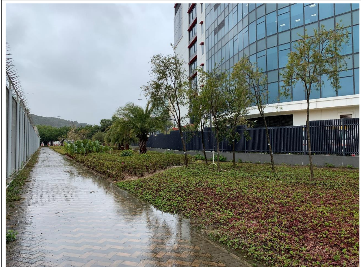
Photo 48: LCSD Area - Zone E
