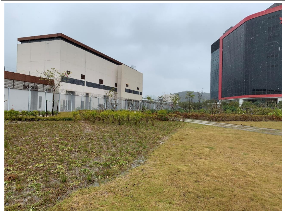
Photo 42: LCSD Area - Zone E
