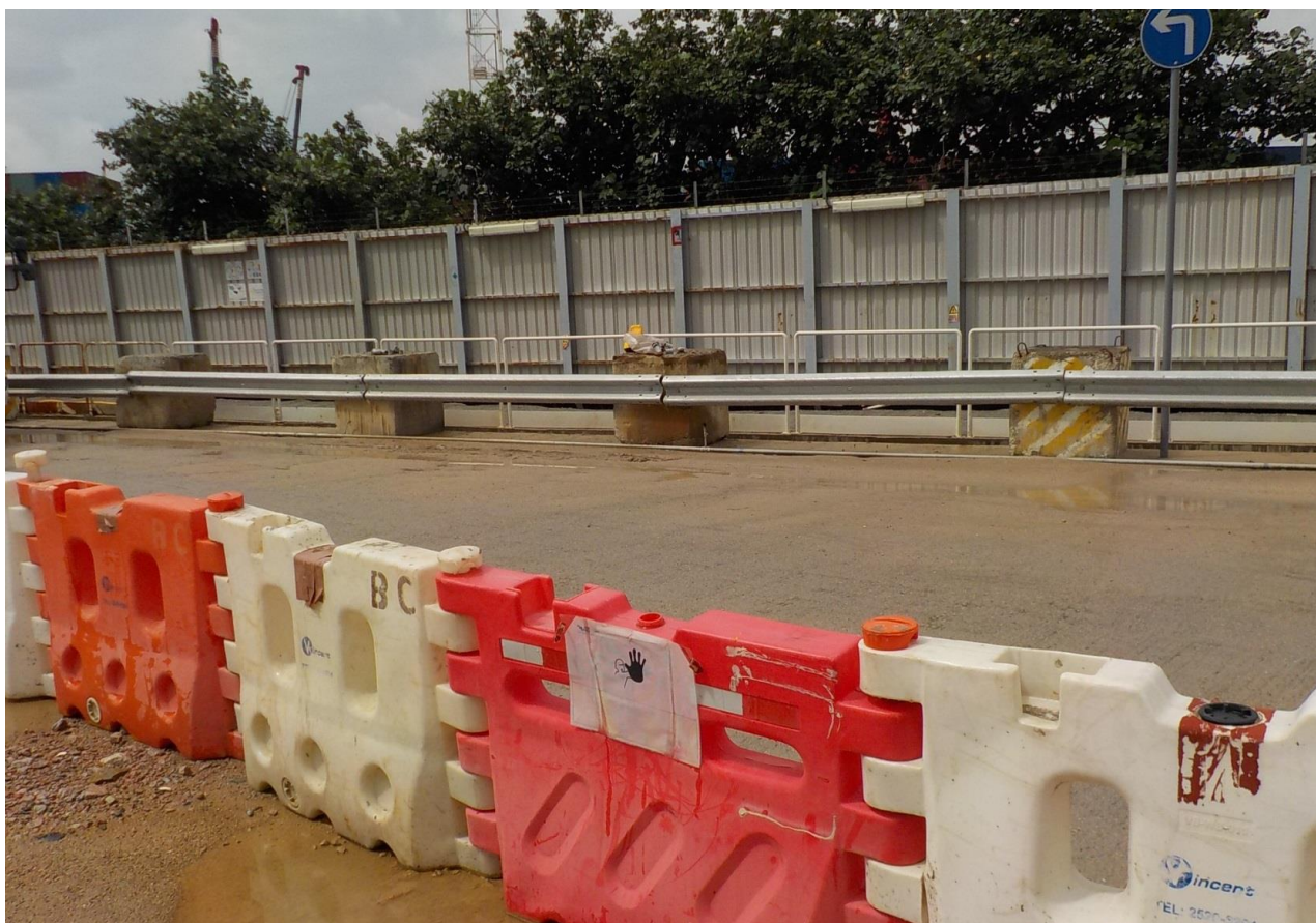
Water spraying was applied to prevent dust.
