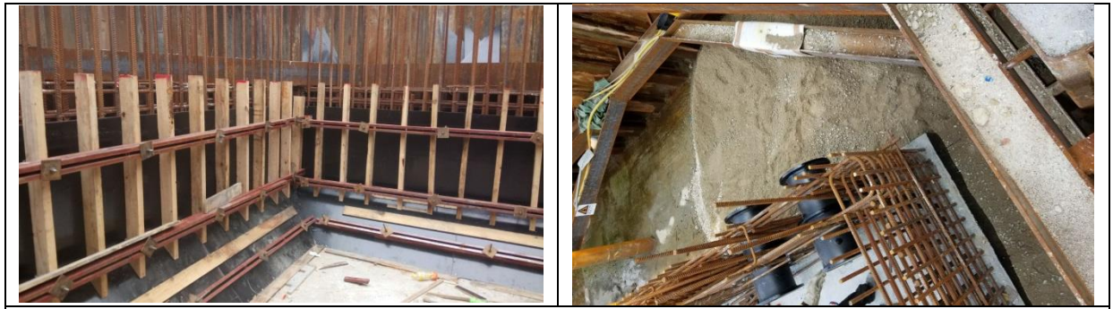
Construction of Pumping Station
