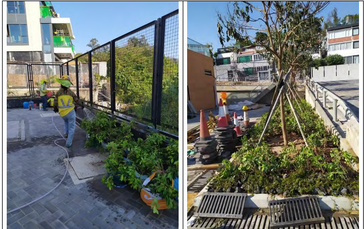
Landscape works and install irrigation
