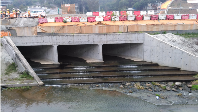
Site photos at I5 during water sampling (Date: 19 February 2016)
