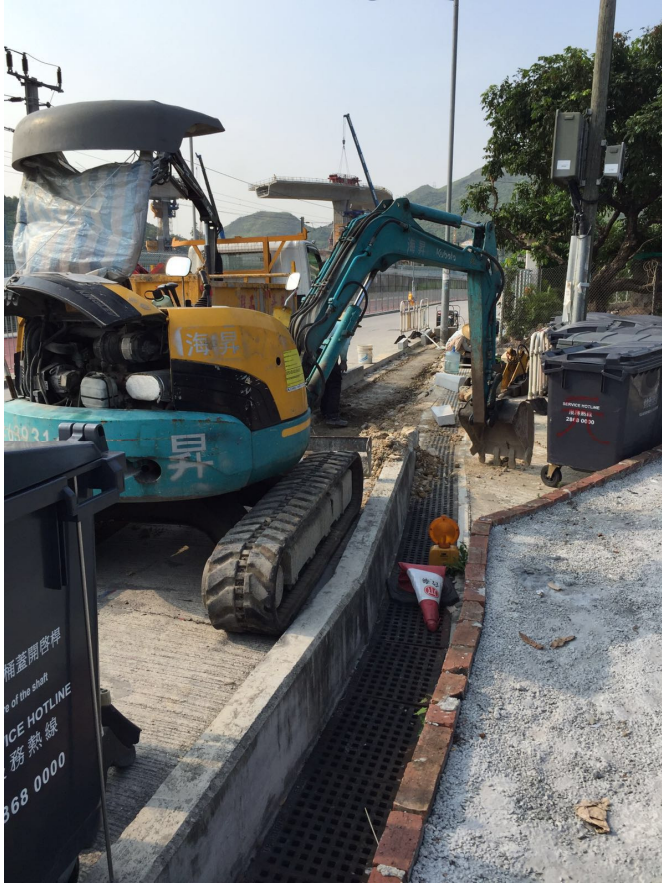
Photo 2: Excavator used for the excavation (Date: 16 May 2016)
