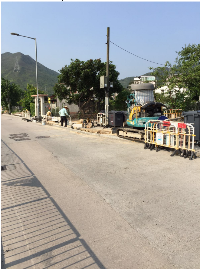
Photo 1: Road Works observed near the Noise Monitoring Station (Date: 16 May 2016)
