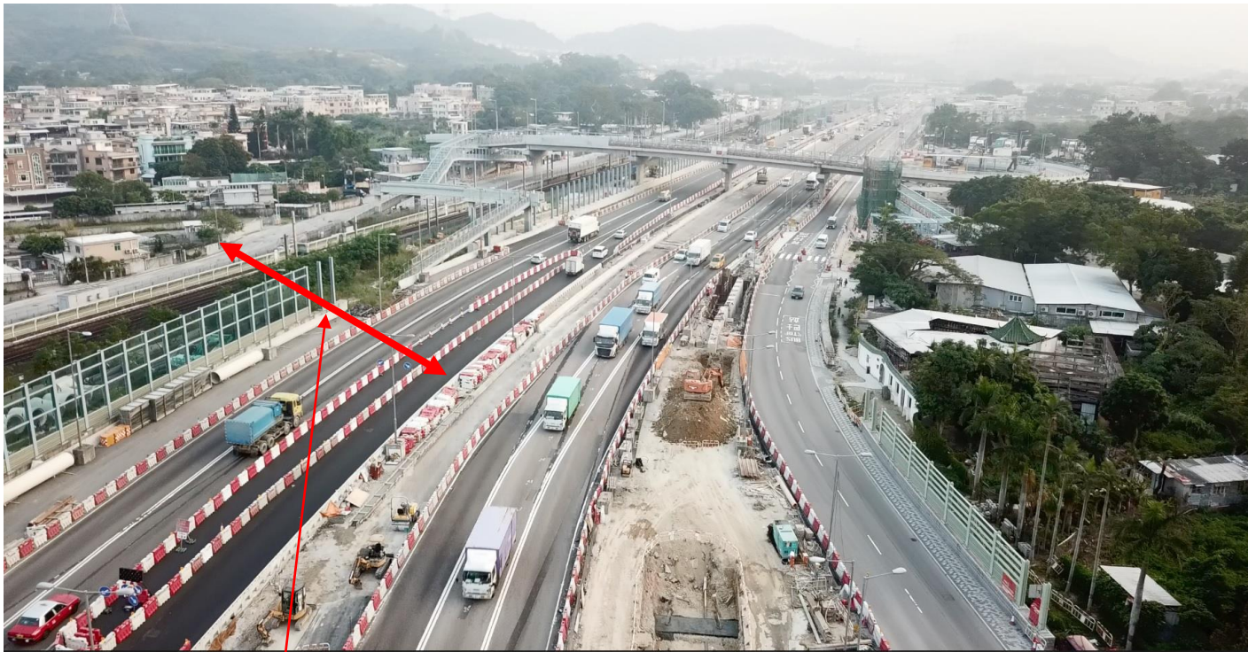
Photo 1: Site photo showing the construction works area and monitoring location (Date: 8 December 2017)
