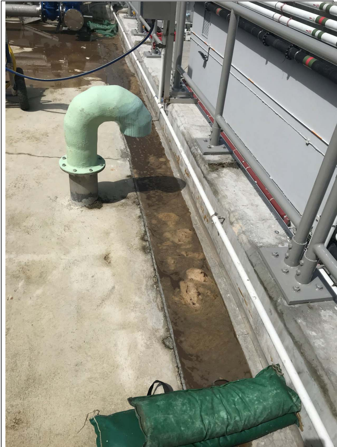
Sand bags were provided for the blockage of rainwater channels.
