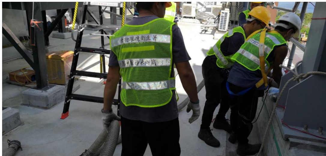
The ACs were being replaced by on site workers.
