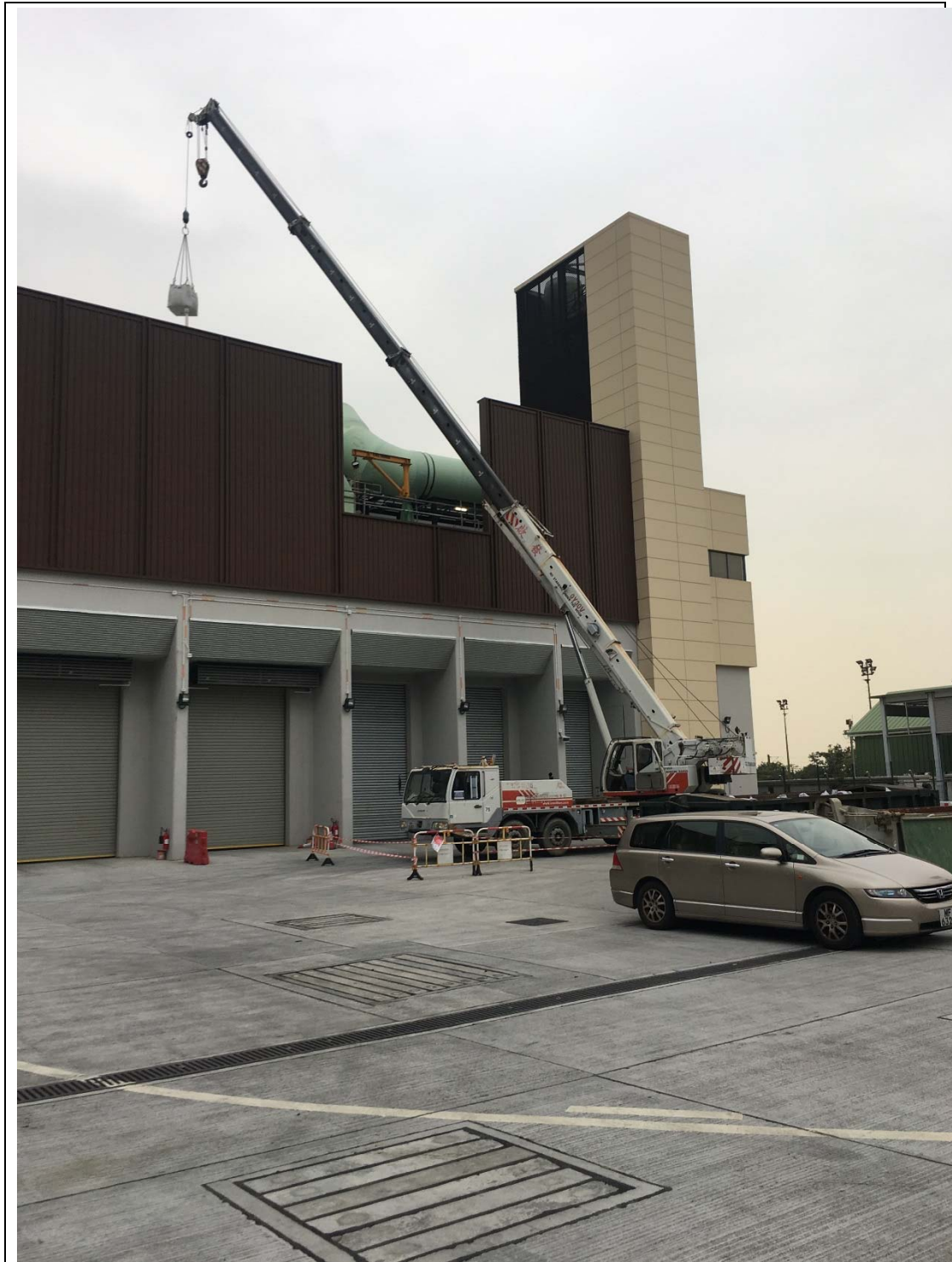
The AC bags were being lifted to roof of the Building 2 and ready for replacement.
