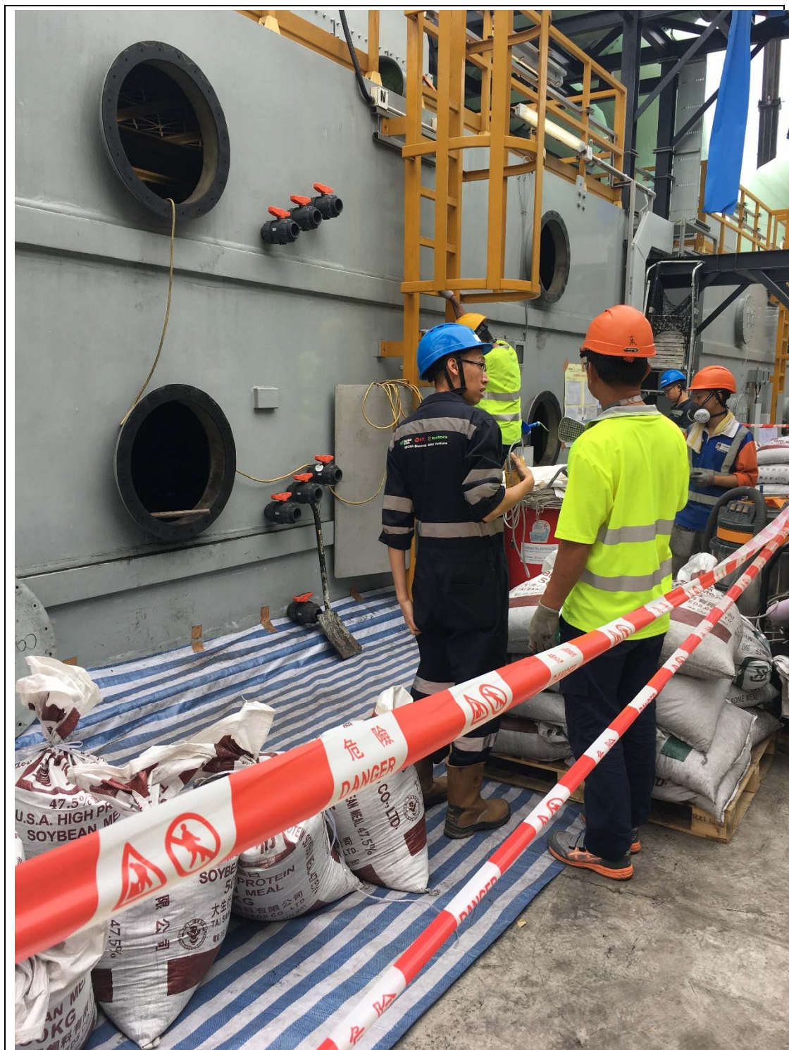
The ACs were being replaced by on site workers.
