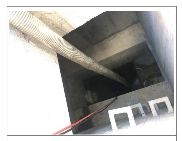
Vacuum tanker was arranged to pump all the residue in the storm water pipeline back to the site wastewater treatment system.
