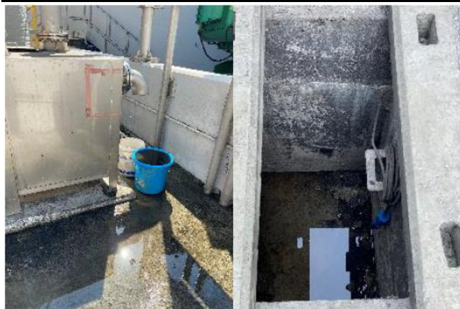
Figure.2 Completed cleanup of tank farm and nearby surface channels
