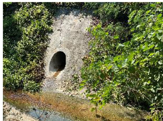
Figure.3 Complete cleanup of nullah
