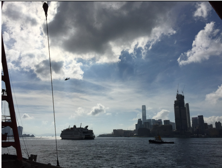
Area near bulk dredging in Victoria Harbour
