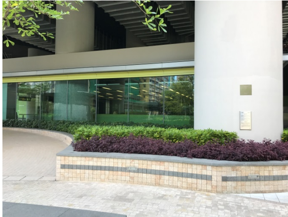
Photo 12 – Vertical greening for HOM structure
