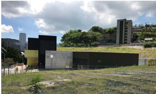
Photo 10 - Backfilled slope with hydroseeded greening
