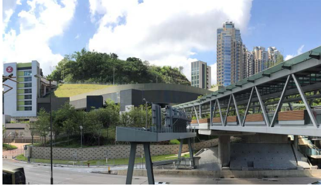
Photo 10 - Backfilled slope with hydroseeded greening
