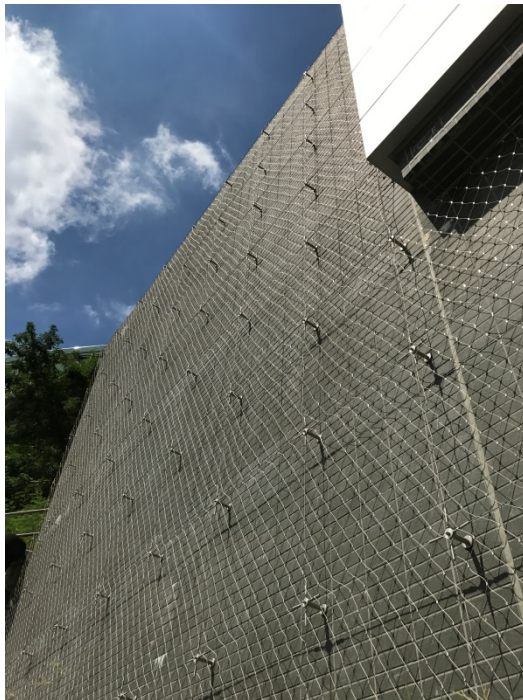
Photo 5 – Metal frame attached to the structure for the climber planting
