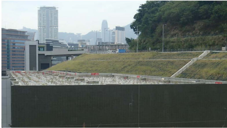
Photo 14 – Temporary roof greening
