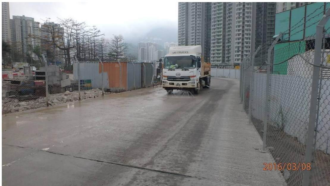
Fig.6 Water truck was assigned for cleaning the haul road.
