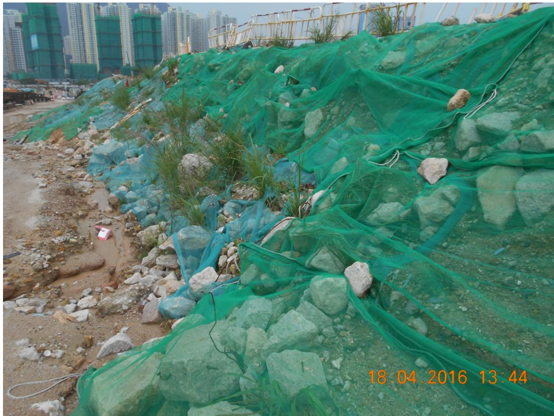
Fig.1 – Inactive stockpile was covered with tarpaulin sheet
