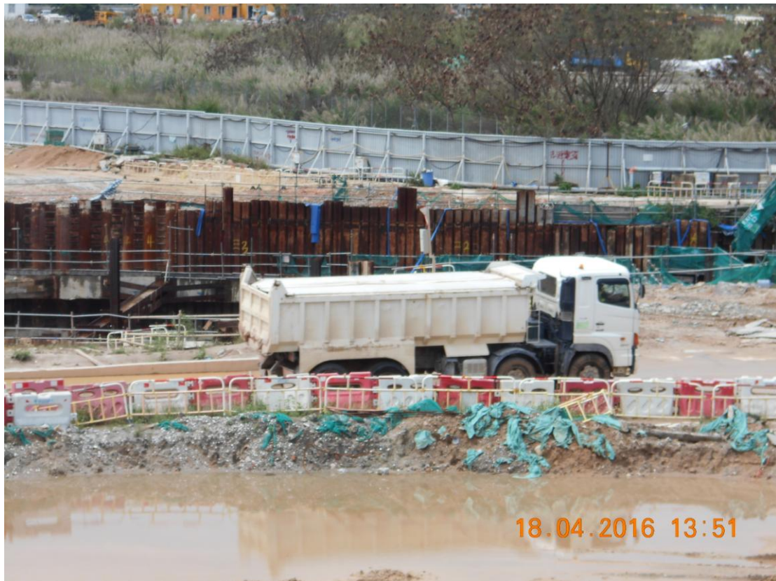
Fig. 5 Construction materials were covered with mechanical cover during the transportation
