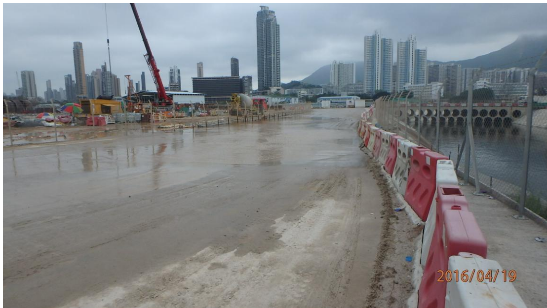
Fig. 6 Water spraying on the haul road was implemented to reduce dust nuisance.
