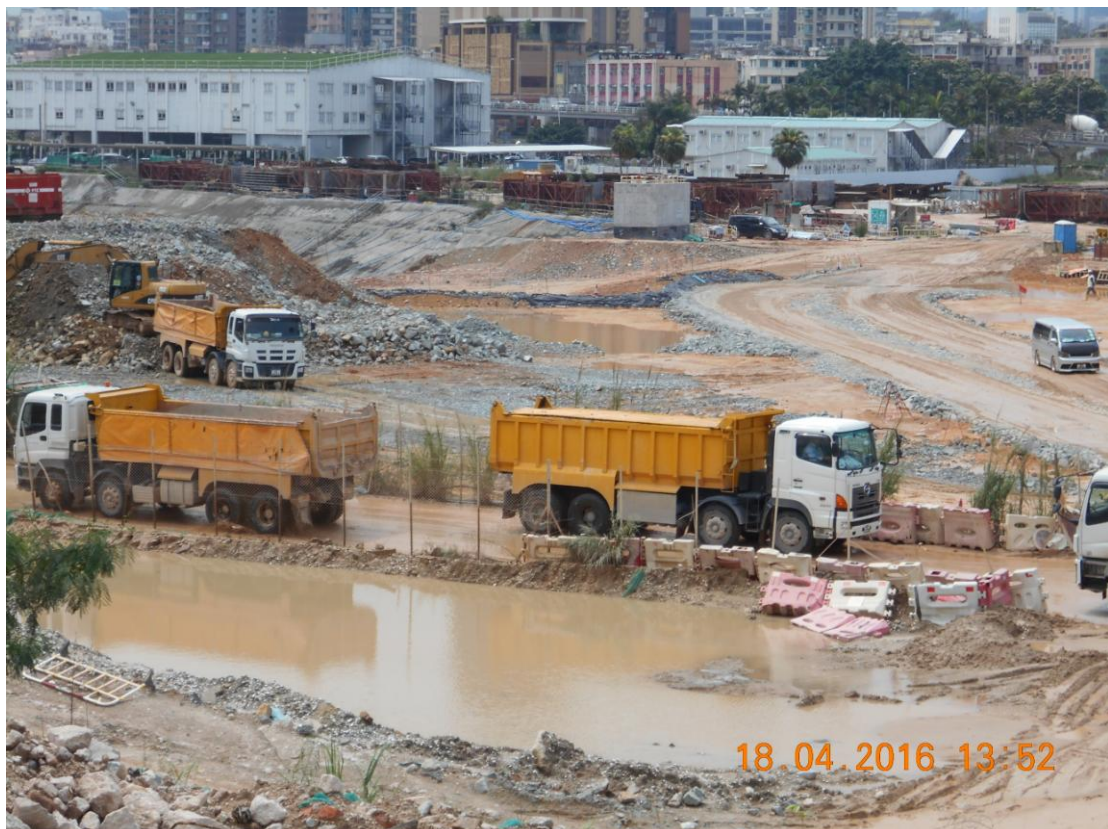
Fig. 4 Construction materials were covered with mechanical cover during the transportation
