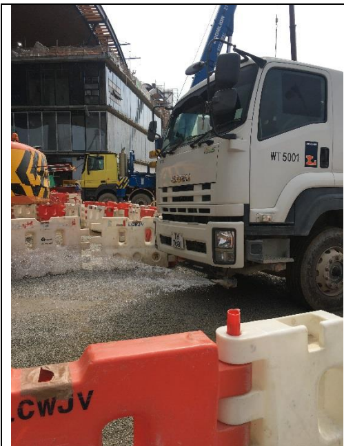
Water truck spray water on haul road (Point C)
