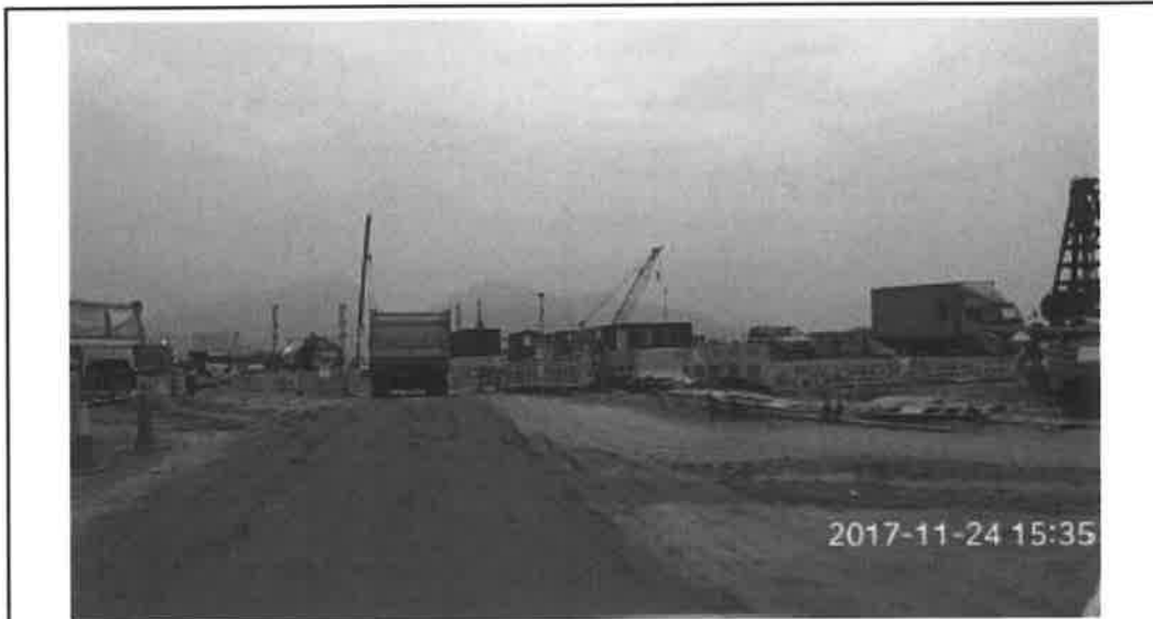
Photo 171124_005 – Watering on the worksite
