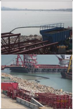
3. Silt curtains provided for marine work areas at Box Culverts C and D.
