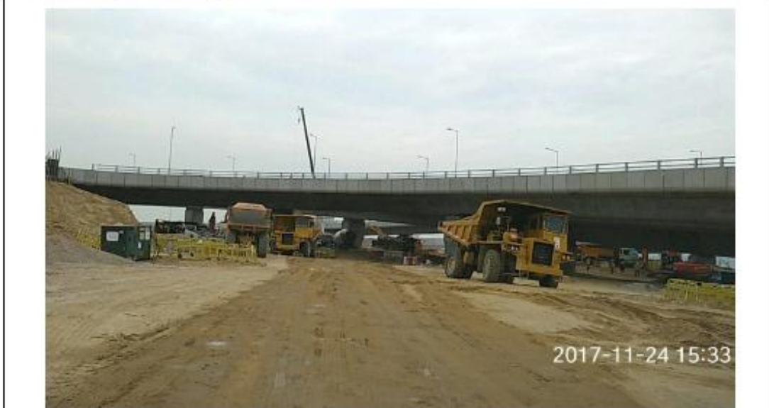
Photo 171124_004 – Watering on the worksite
