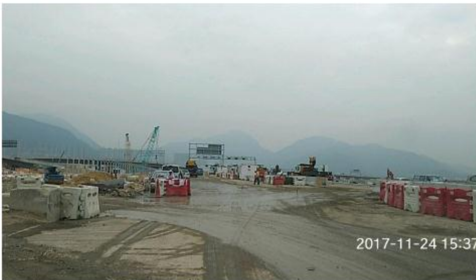
Photo 171124_006 – Watering on the worksite
