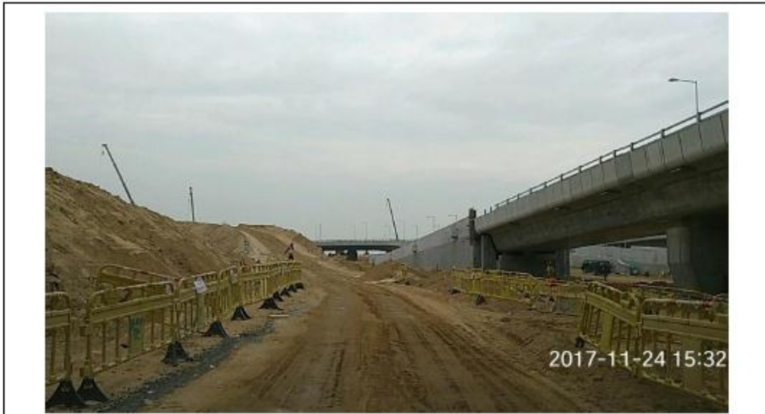
Photo 171124_003 – Watering on the worksite
