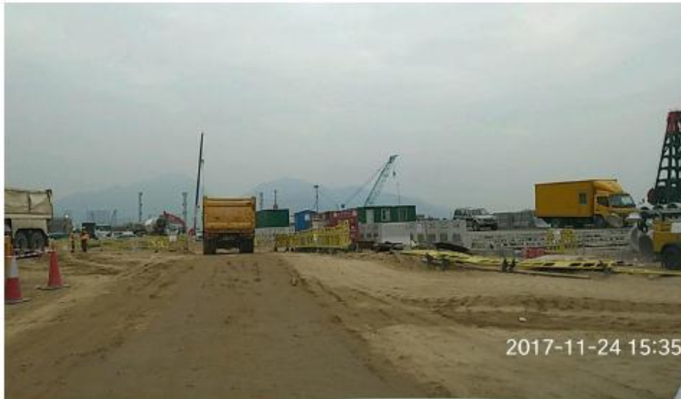
Photo 171124_005 – Watering on the worksite
