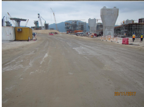
1c. Water spray provided for haul roads in the HY/2013/04 site area (near Bridge D12). No fugitive dust generation was observed.
