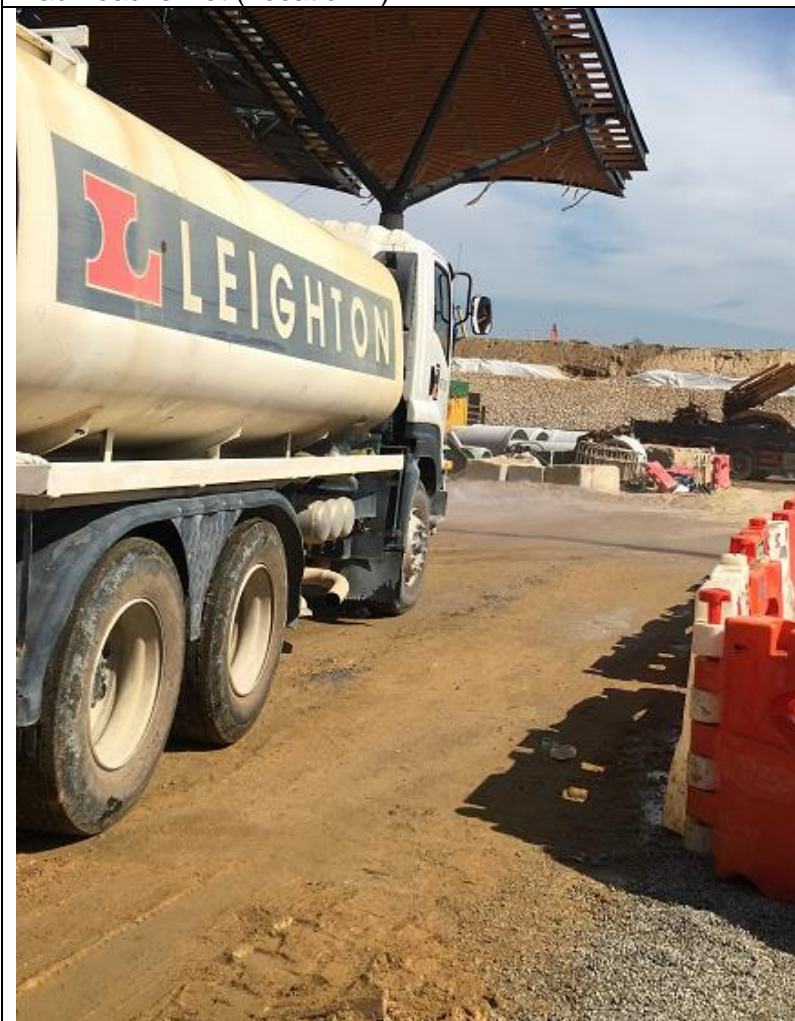
Water truck spray water on haul road (Location 2)
