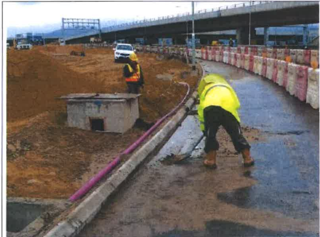
Photo 2.5 – Manpower was provided to clean-up the accumulated mud/slurry along the roadside
