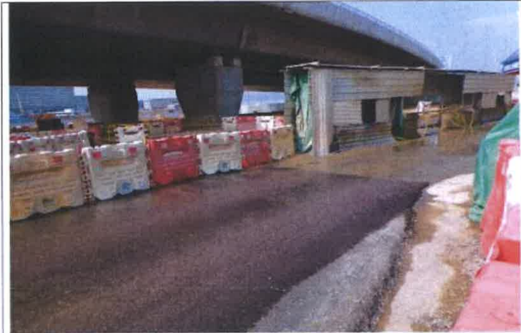
Photo 1.6 – The road section between washing facilities and site exit on 08 February 2018
