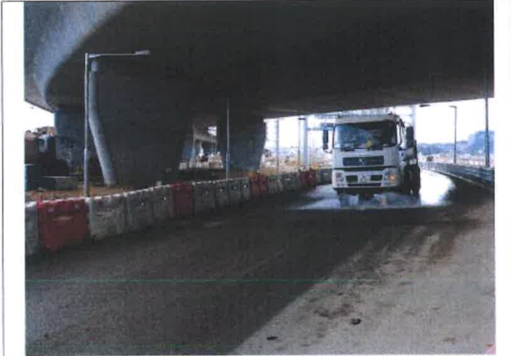
Photo 2.3 – Watering truck was provided to water the road section between washing facilities and site exit
