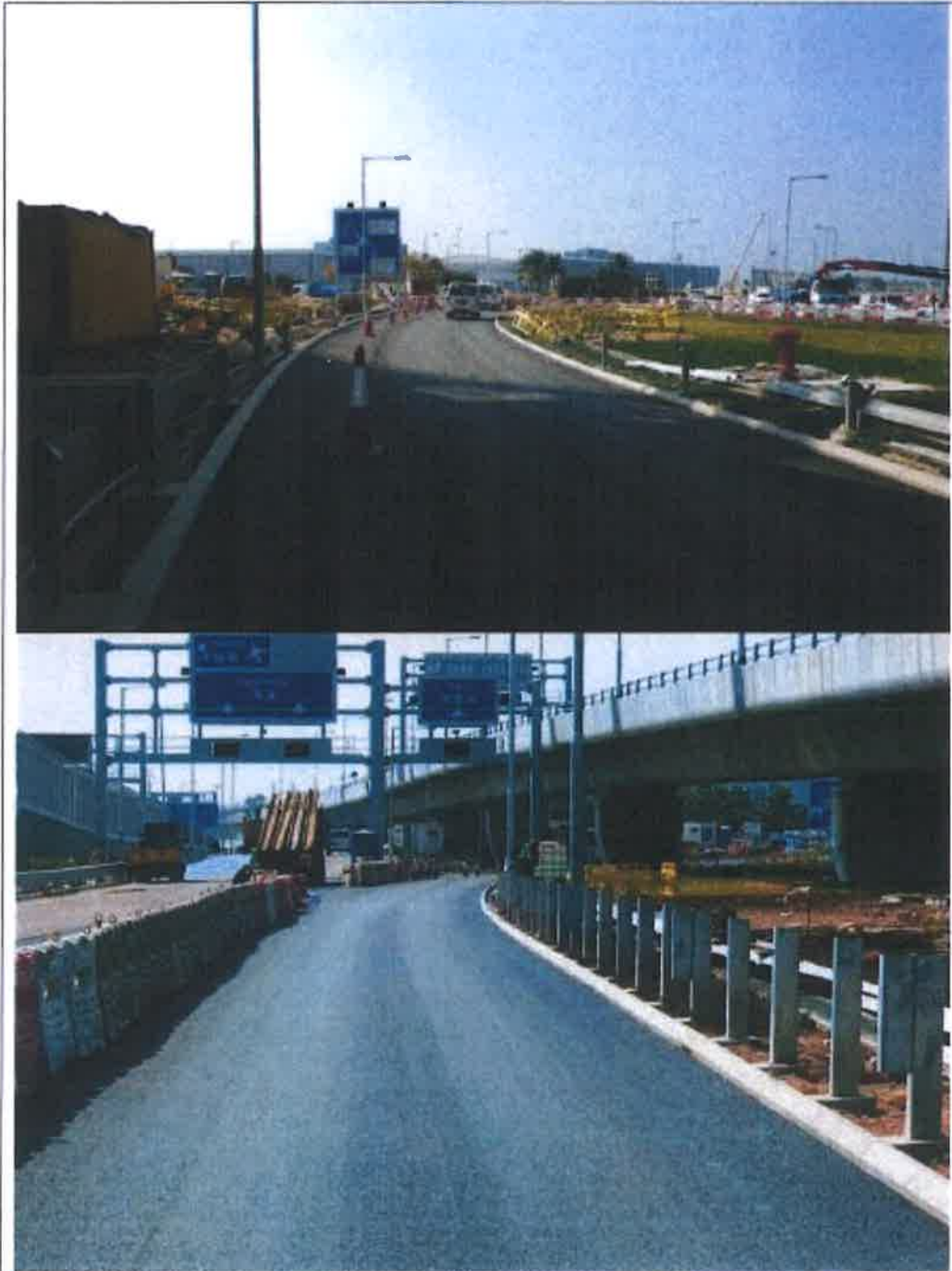
Photo 1.8 – The road section between washing facilities and site exit on 12 February 2018
