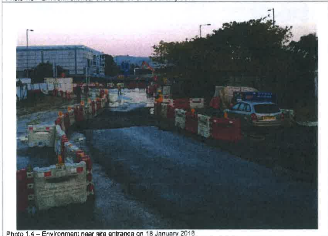
Photo 1.4 – Environment near site entrance on 18 January 2018
