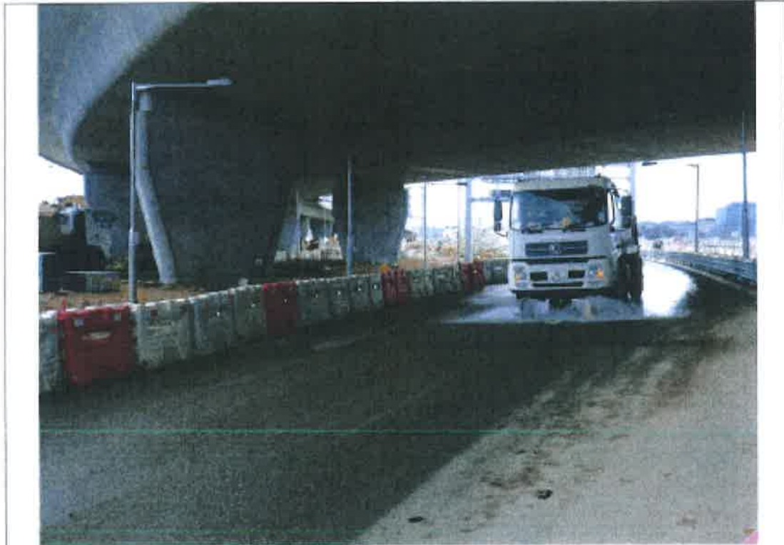
Photo 2.3 – Watering truck was provided to water the road section between washing facilities and site exit
