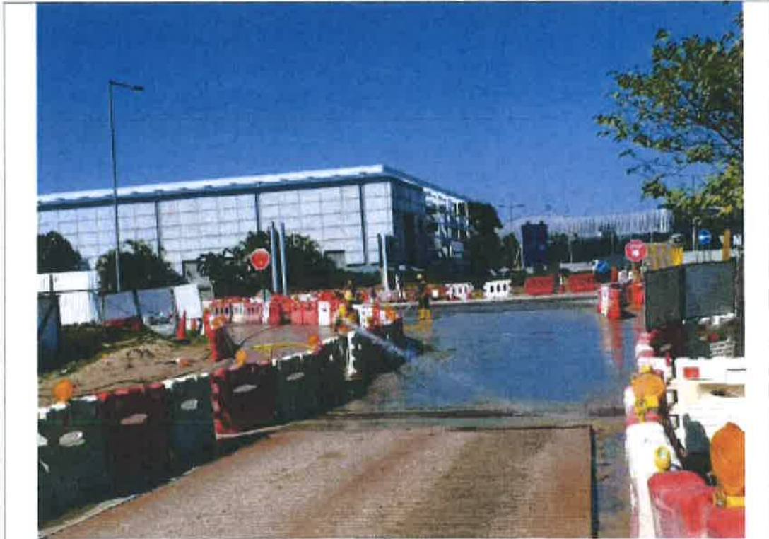
Photo 1.3 – Environment near site entrance on 12 January 2018
