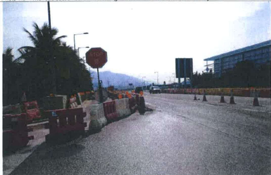
Photo 1.7 – Environment of East Coast Road near site exit on 08 February 201
