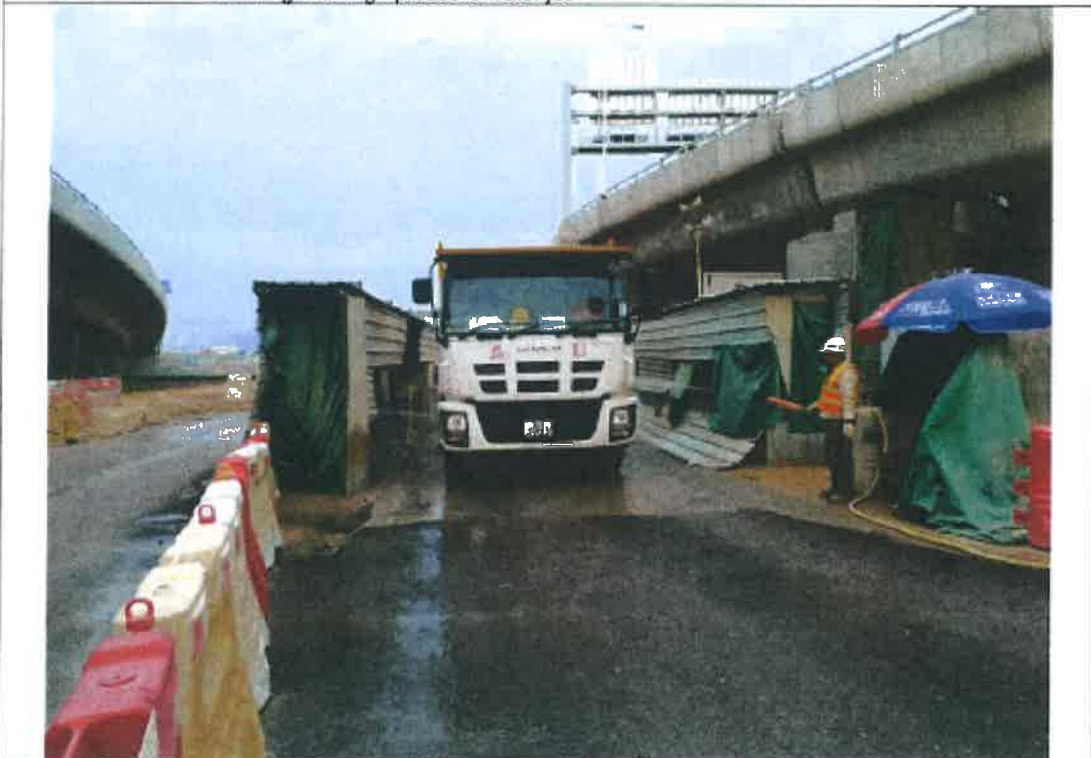
Photo 2.2 – Manpower was provided for stopping the vehicle when passing the washing facilities
