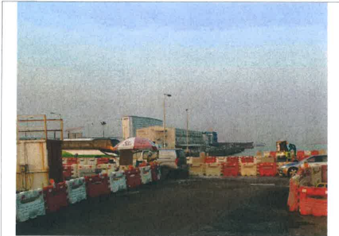
Photo 2.1 – Further washing with high pressure water jet
