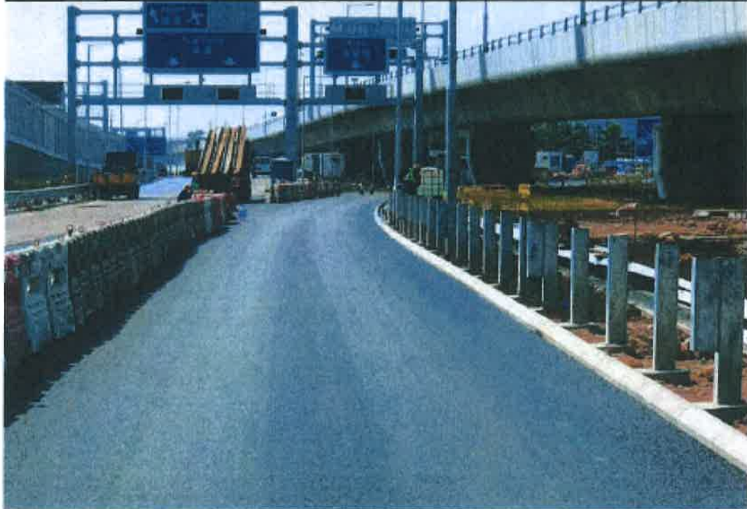
Photo 1.8 – The road section between washing facilities and site exit on 12 February 2018
