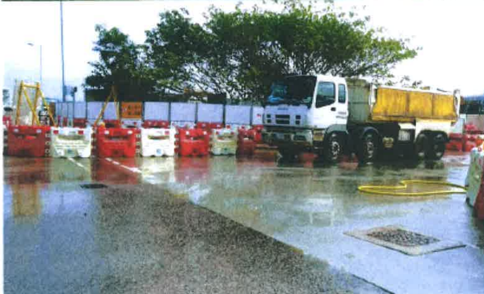
Photo 1.1 – Environment near site entrance on 10 January 2018
