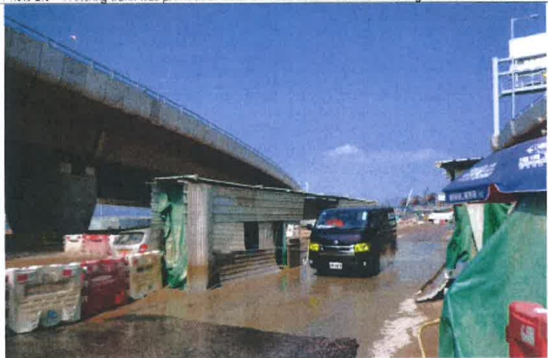
Photo 2.4 – Wheel-washing facilities with high pressure water jet
