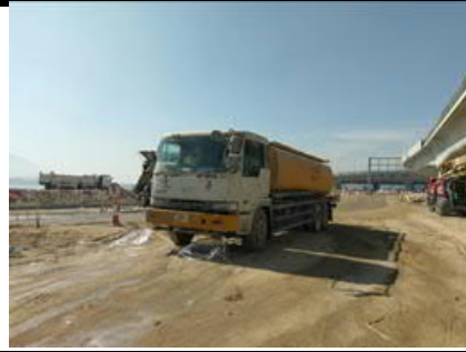
4b. Subsequent follow-up action by Contractor: provision of water spray.
