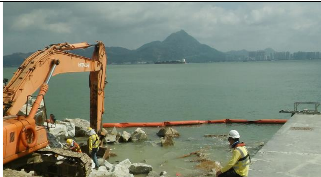
Photo 3 | Construction of seawall
