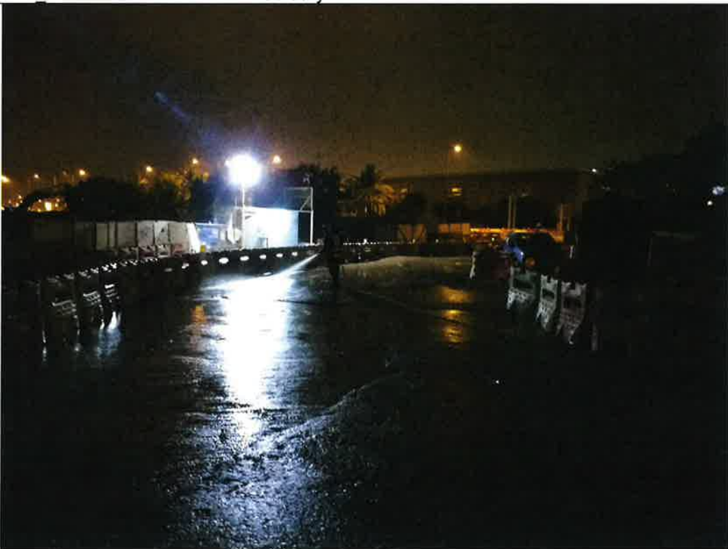
Photo 180208_002 – Photo taken on 29 January 2018 at the site exit
