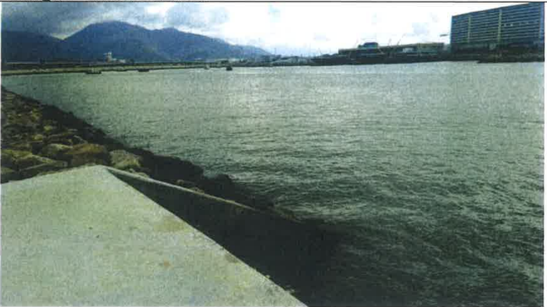
Photo 180625_002 –Box Culvert A on 25 June 2018
