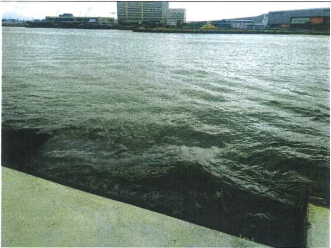
Photo 180625_001 –Box Culvert A on 25 June 2018
