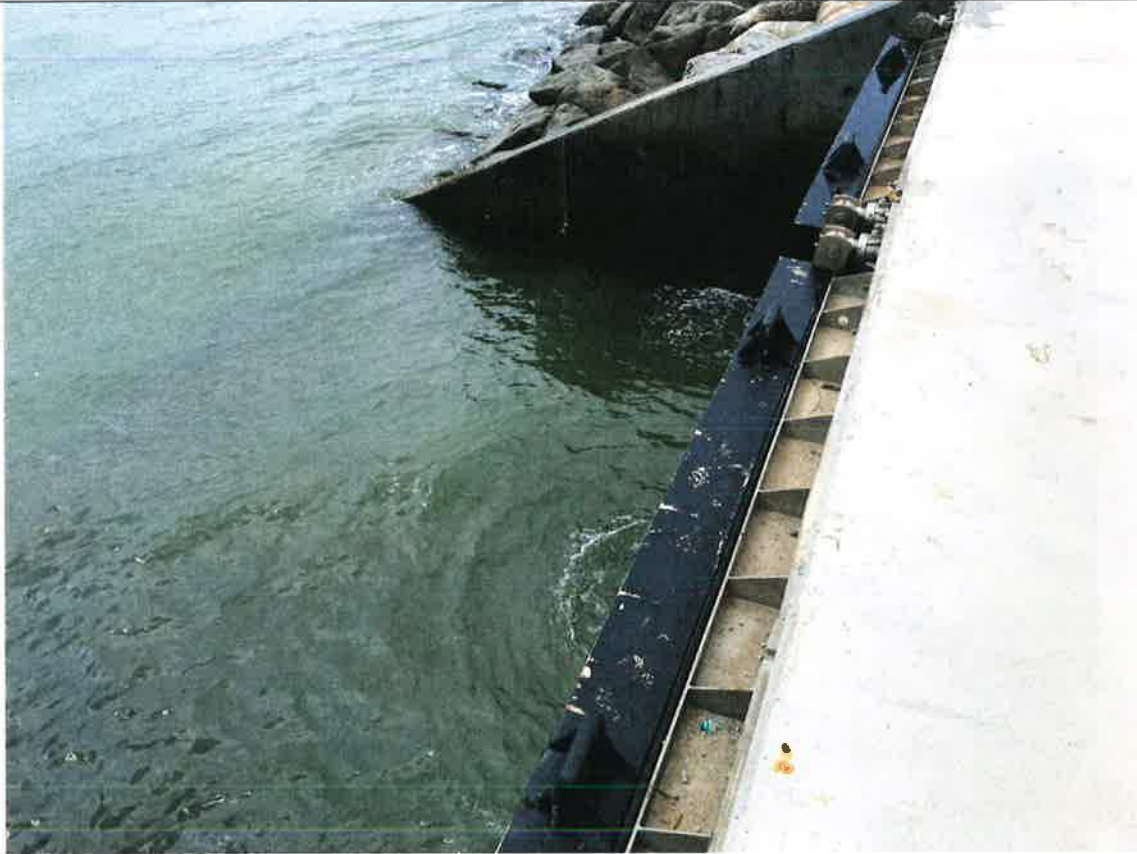
Photo 180627_001 –Box Culvert A on 27 June 2018
