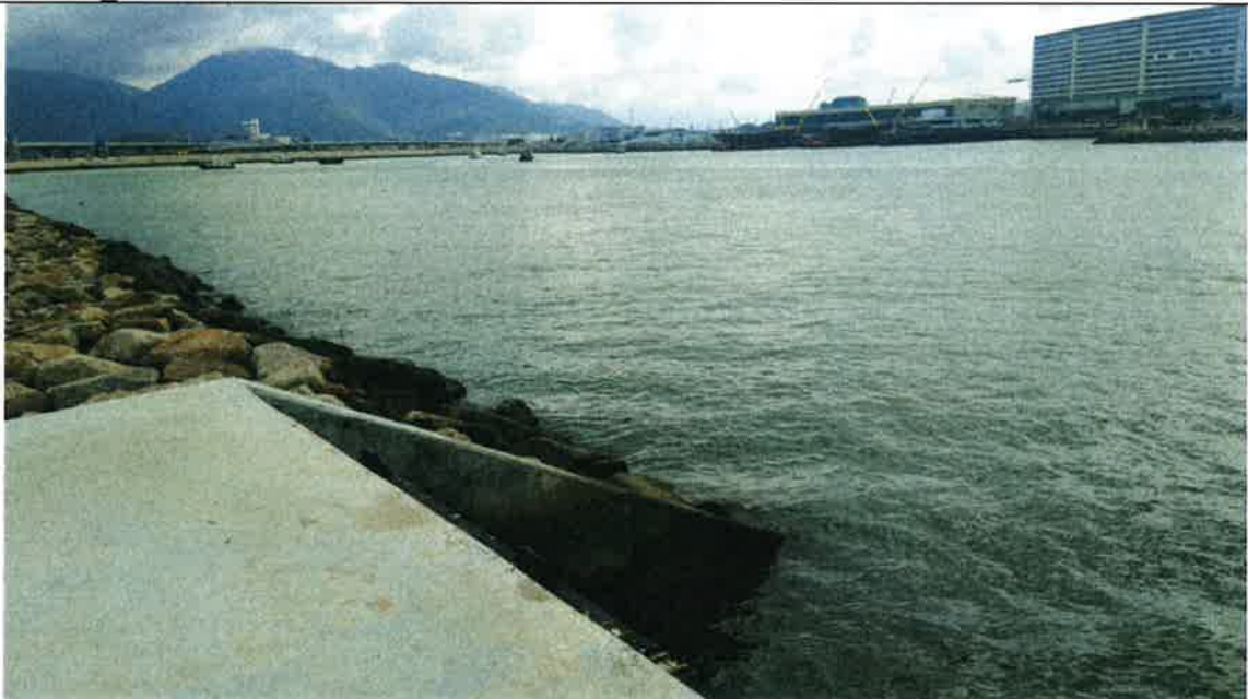
Photo 180625_002 –Box Culvert A on 25 June 2018
