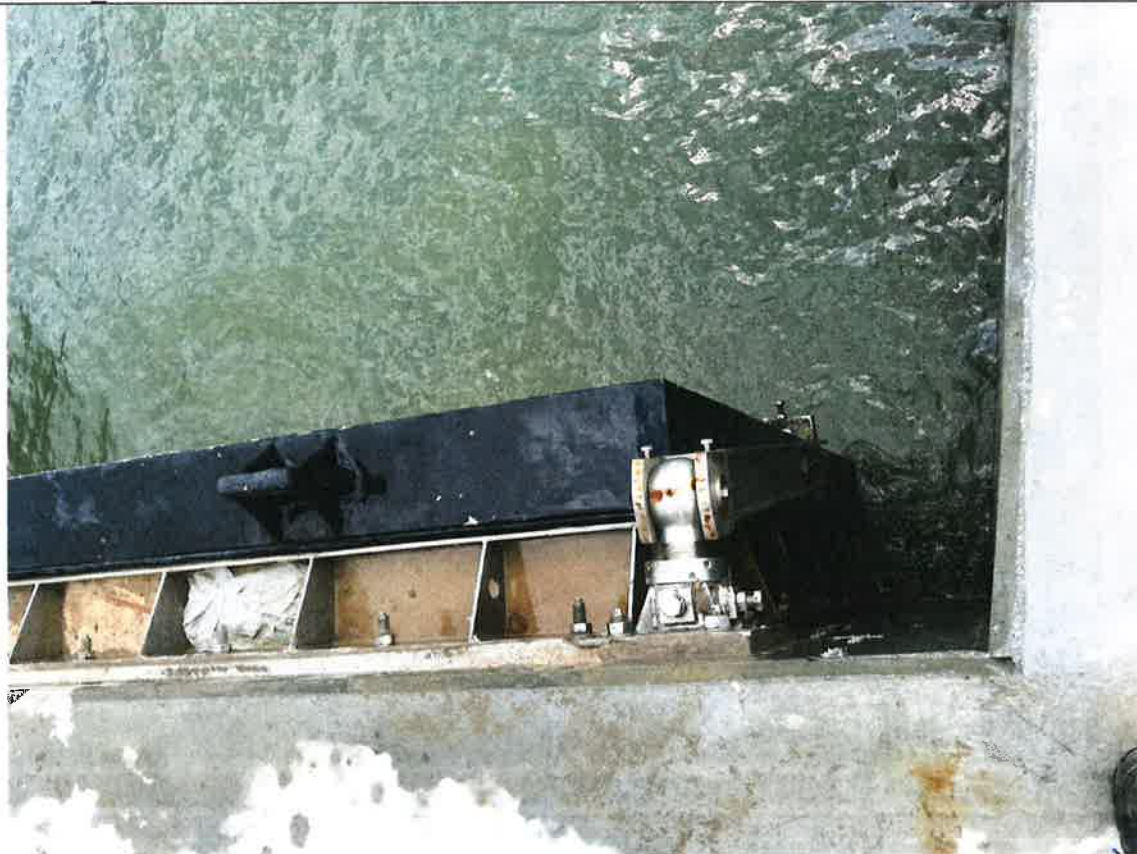
Photo 180627_002 –Box Culvert A on 27 June 2018
