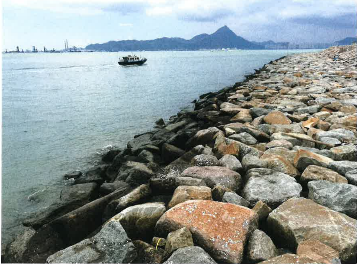
Photo 180627_003 – Open sea near Box Culvert A on 27 June 2018
