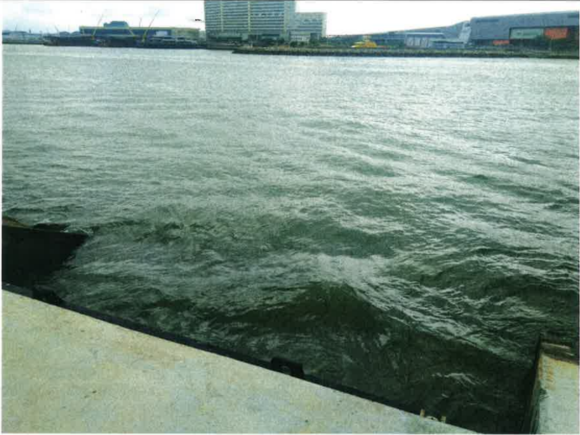
Photo 180625_001 –Box Culvert A on 25 June 2018
