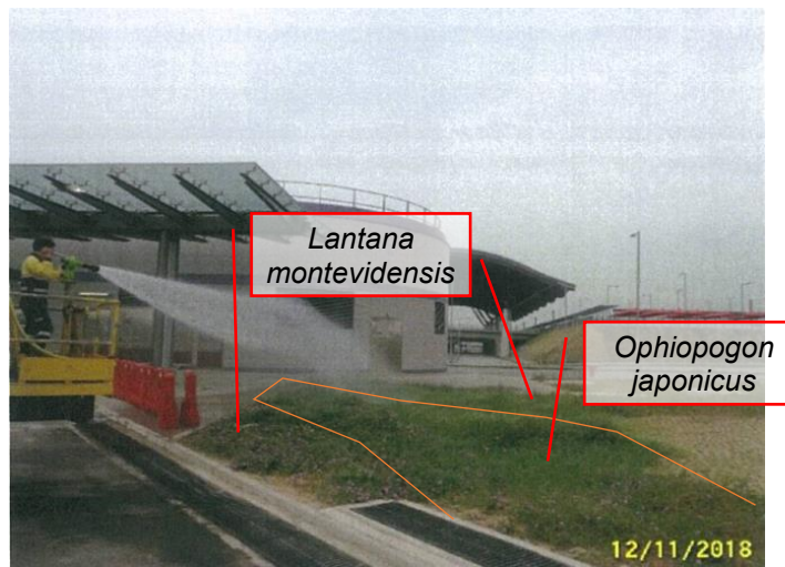
Building 025 at-grade planting (Photo 7 and Photo 8)
